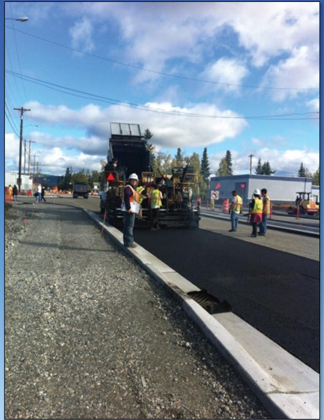
A paving crew from H C Contractors Inc. lays asphalt on the Illinois Street project this summer.
